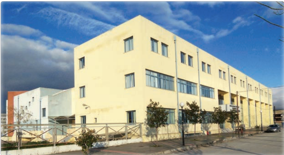
■ PRD Building: South-east face
