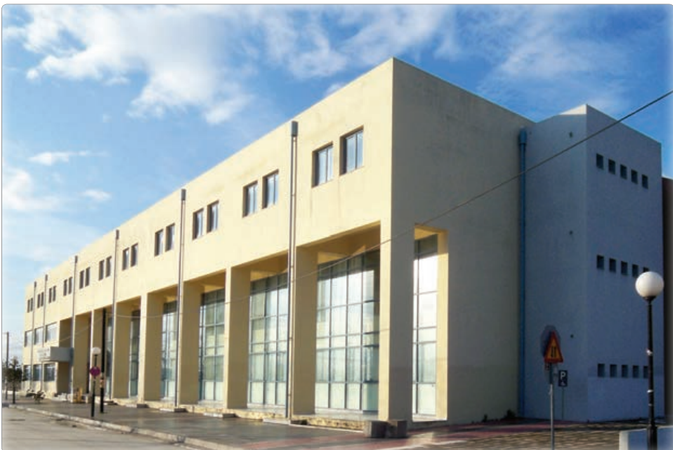
■ PRD Building: North-west face
