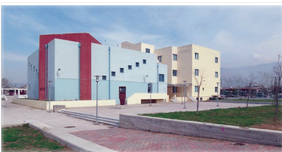
■ PRD Building: North-east face
